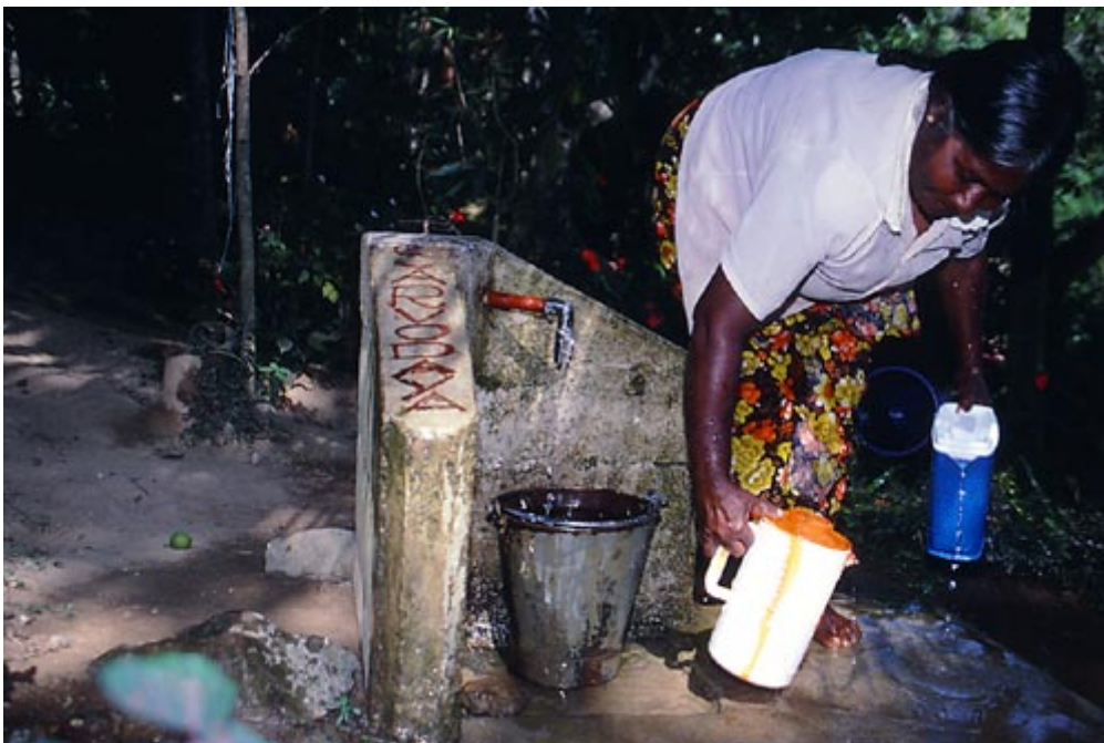
A public standpipe in Menderipitiya's water supply
