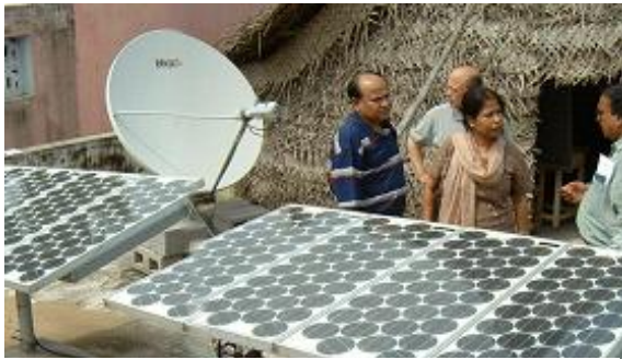
Satellite like for a local area network and solar cells providing uninterrupted power for the network (Southern India)
