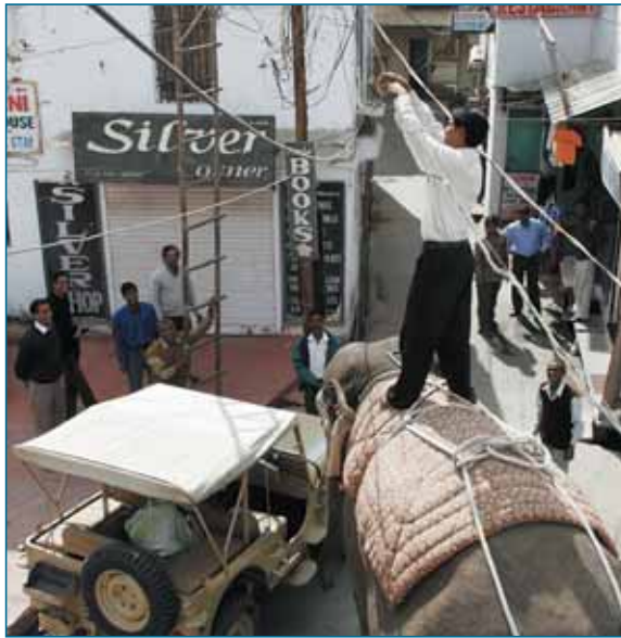
A man attempts to fix a wiring problem while standing on an elephant, Udaipur, Rajasthan, India QILAI SHEN | PANOS PICTURES
