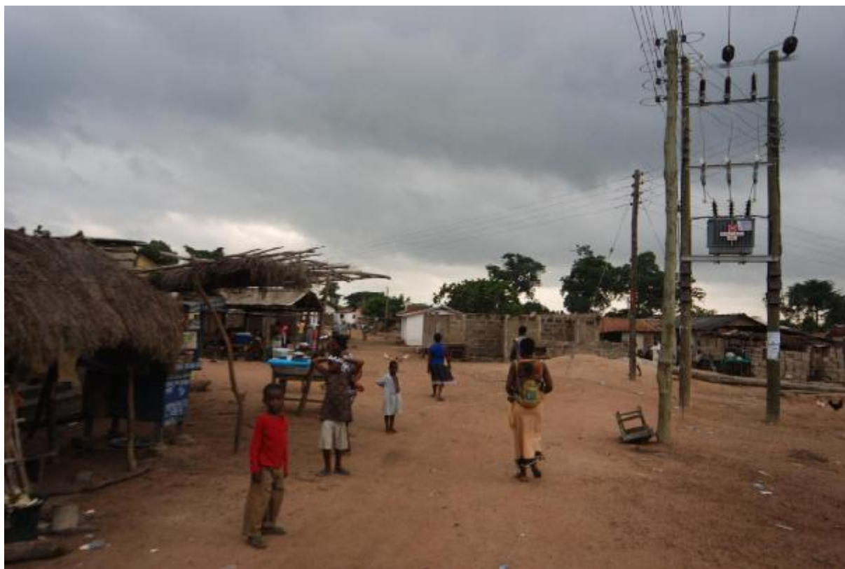
Ghana’s rural electrification stands at the beginning, but is being pushed by the government.
